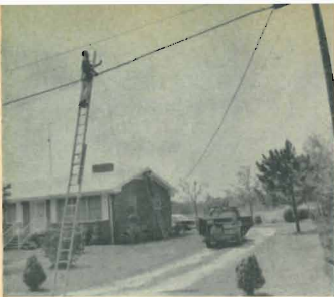
Lineman installing tap-off connecting subscriber's home to cable.
